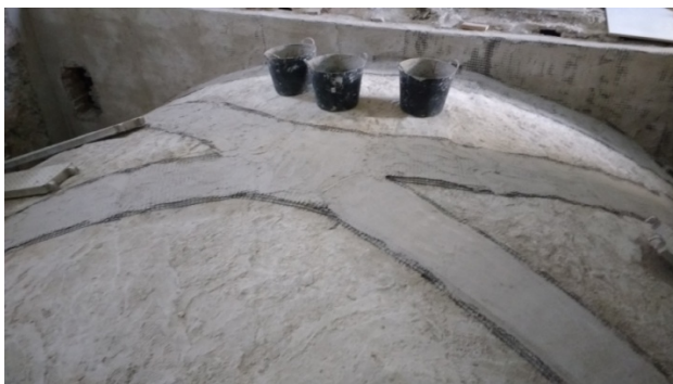
Figure 2: Reinforcement with Planitop HDM and fiberglass Mapei
