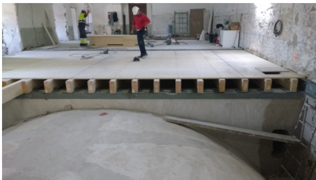
Figure 3: Reinforcement on wall ribs
