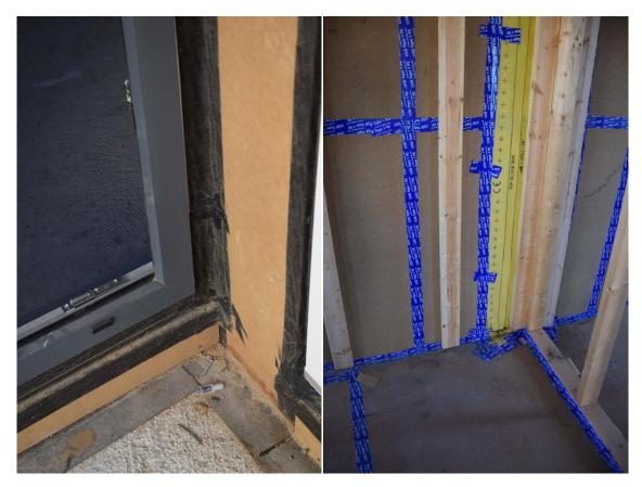
**Figure 5.** Lacquered aluminium carpentry joined to the exterior pavement. Airproof sealing and waterproofing with EPDM (left). Interior partitions and enclosure with tape sealing, type Riwega USB Tape 1 PE (right).
