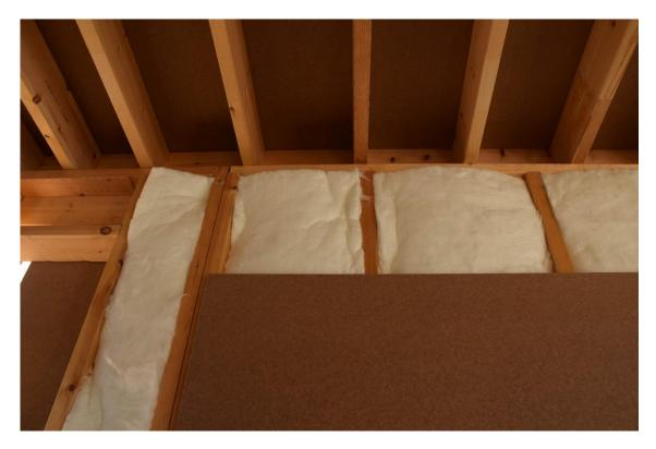
**Figure 4.** Wooden structure and Superpan Tech 15 mm board partitions with 148 mm mineral wool thermal insulation.
