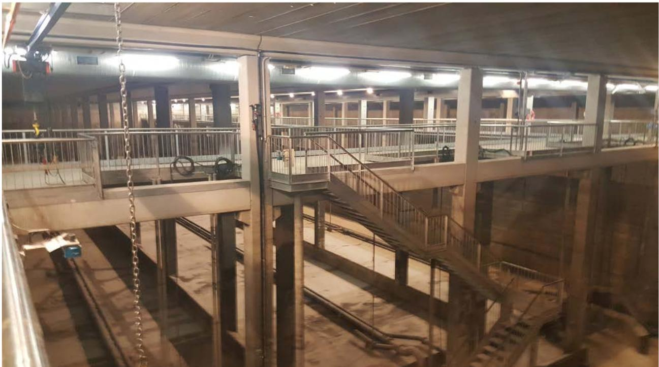
**Figure 2:** The inside of the anti-pollution tank is shown. *Source: the Authors.*
