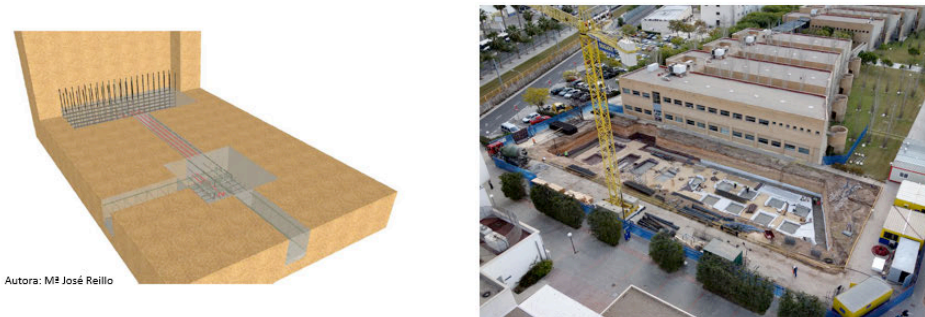
Fig. 6. Simulated 3D image. Superficial foundation and aerial view of a construction building. Emplacement of equipment, installation and auxiliary resources.
