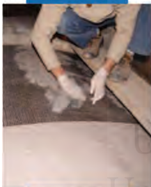
Positioning of Mapegrid B 250
