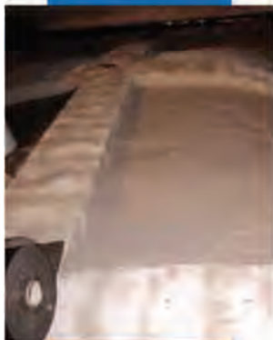
Application of the first layer of Planitop HDM Restauro
