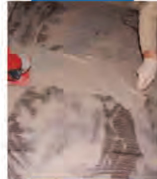
Application of the second layer of Planitop HDM Restauero
