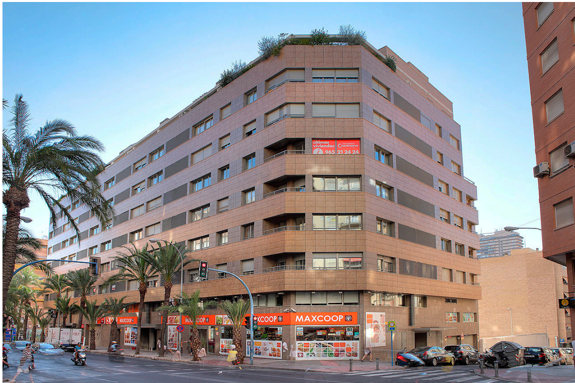
Figure 7. The northeast view of the building.
