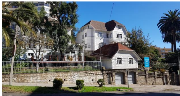
Fig. 2: Image of the Building Studied, Located in Traslaviña 450 Street in The City of Viña del Mar. It Currently Serves as the Center of Advanced Studies for the Universidad De Playa Ancha.
