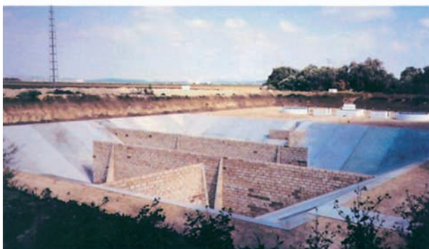
Fig. 8.- Settling-basin with walls to improve deposition of suspended solids.
