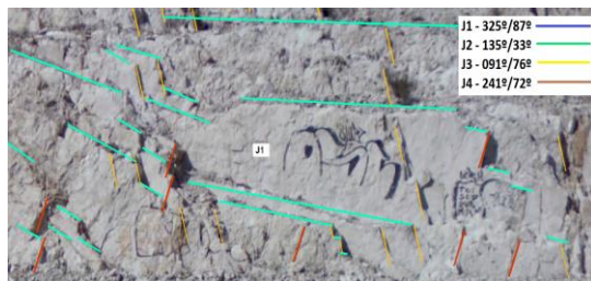
Fig.4: Plot of the discontinuity sets identified by the LiDAR.
