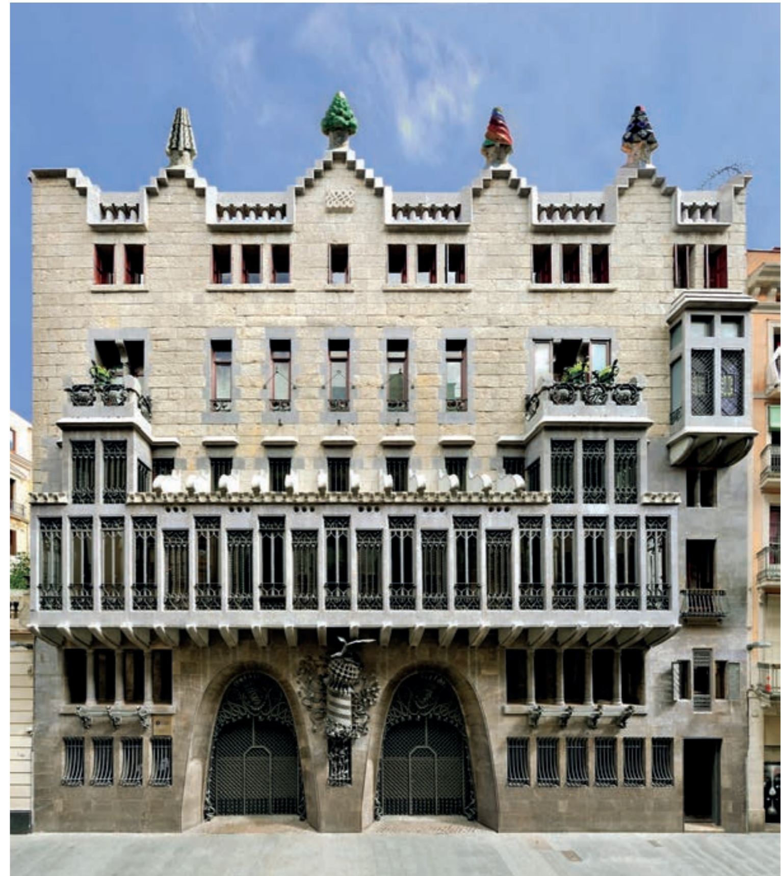
Palau Güell, in Barcelona. Main Façade. This color photograph is the same as the cover of the book The Güell Palace (2013). This sophisticated picture, which is from such a frontal perspective, is a good example of the uses of new technologies in architectural photography. (Photo: ©Montserrat Baldomà, April 2012. Tiff digital file. SPAL Archives.
