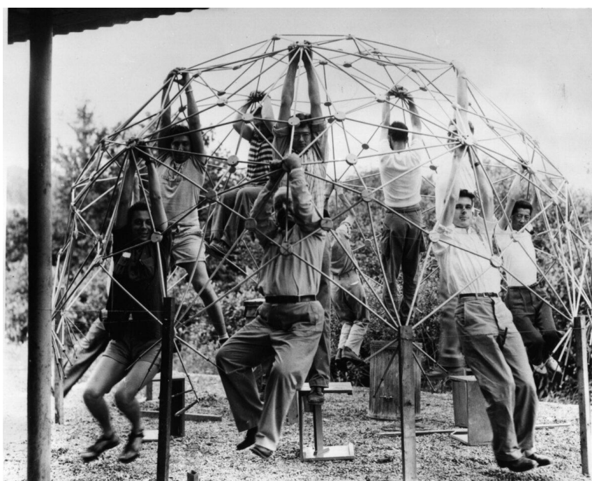
Figure 2. Demonstration of the strength of the dome; Buckminster Fuller and students hang from sections of the dome [41].
