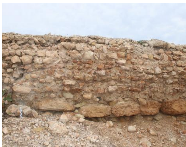
Figure 13: Photography of the back of the East wall. The rudus, the calcarenite blocks and the masonry of the wall are observed.
