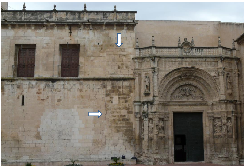
Figure 6. Northeast façade of the church.
