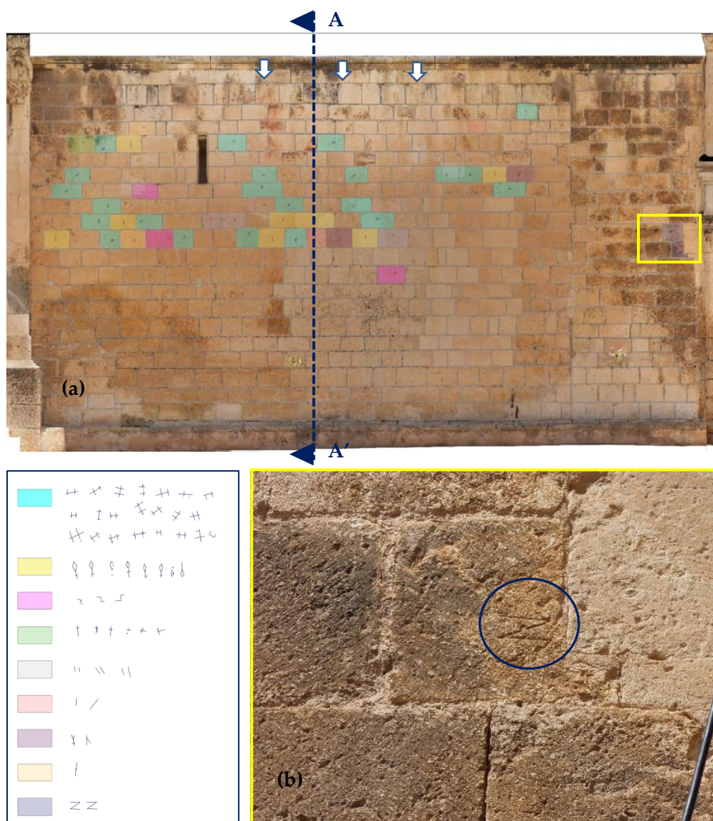
Figure 7. (a) Northeast façade of the church with ashlar coloured according to the type of stonemason marks, in the attached table. (b) Inside the circle detail of a mark that coincides with those of the Gothic church of Jávea (Alicante).
