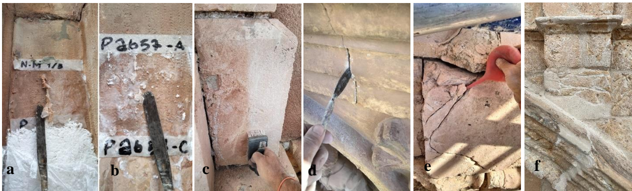
Figure 11. Different aspects of pre-testing of crack cleaning and crack sealing.
