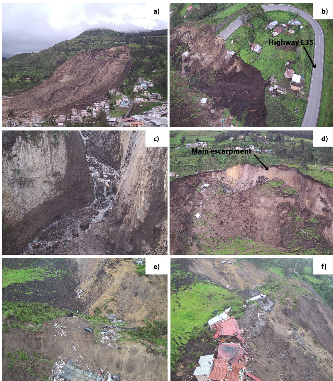
Fig. 4 Evidence of the Alausí landslide on March 26, 2023. a Rupture zone and rotational displacement. b Destroyed 1.2-km section of highway E35. c Quebrada el Tingo. d Main escarpment of the landslide with outcrops of three lithological units. e Homes and vehicles affected. f Total collapse of houses in the body of the landslide
