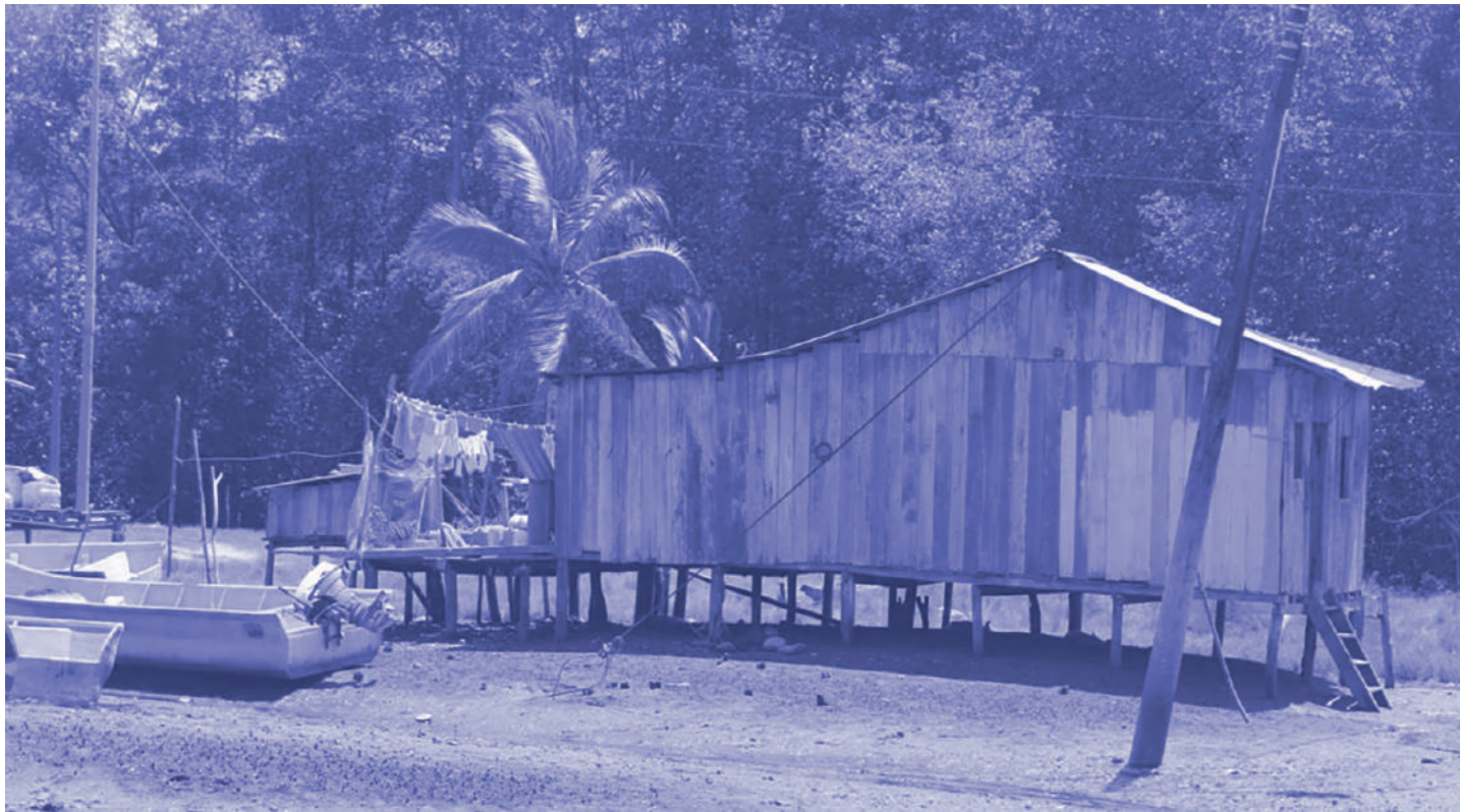
Fig.6 – Typical house. Author source.
