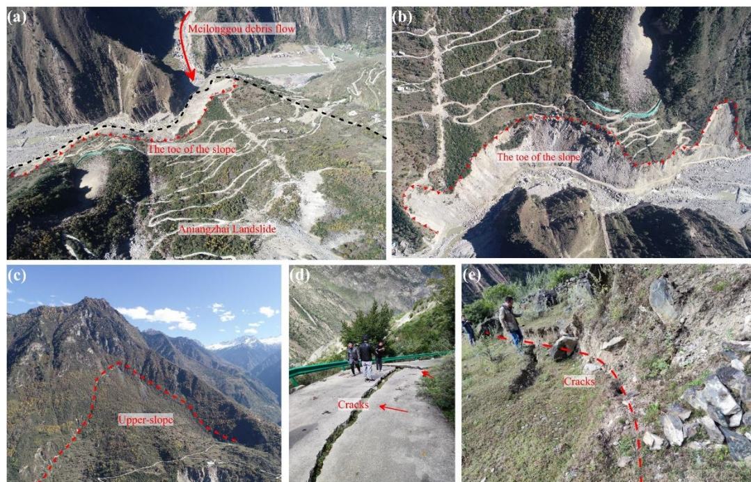
Fig.2 Field work photos of Aniangzhai landslide. (a) and (b) show the toe of the slope collapse related to Meilonggou debris flow. (c) Upper-slope area of Aniangzhai landslide. (d) (e) Tension cracks. The approximate locations of the pictures are shown in Figure 1.
