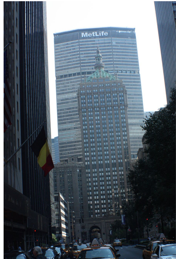
Fig. 25 The MetLife Building threatens the presence of the neoclassical building
