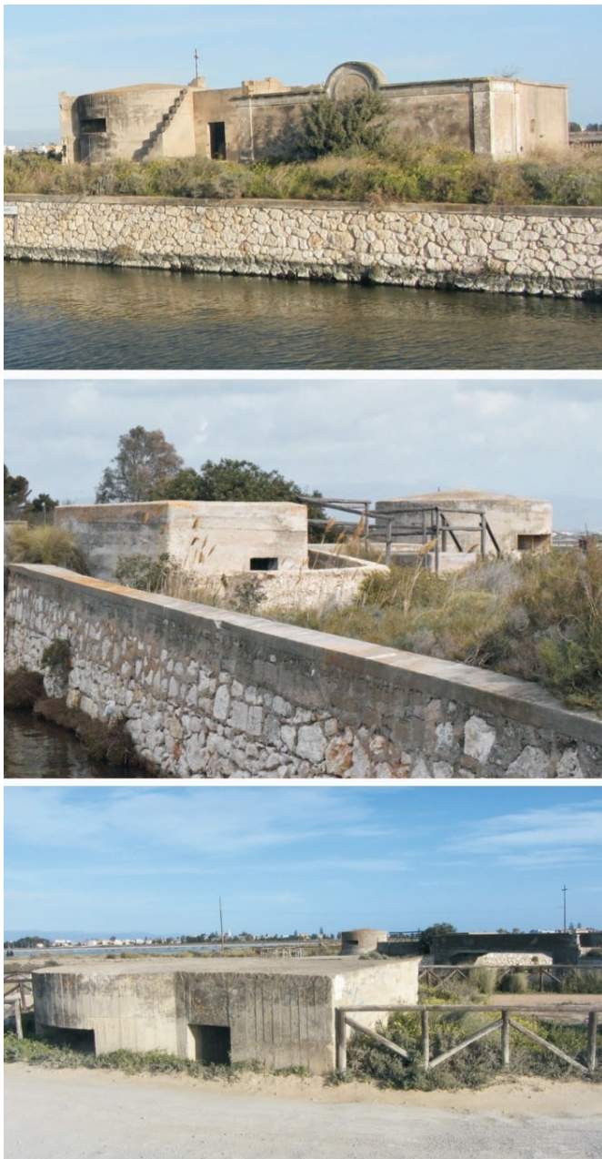
Figure 13. Sector 2. (Top) Bunker modified as a water tank (2a to reach a complete mimemisis with the landscape), (Medium) circle + square connected through a vaulted passage (2b) and (Bottom) bunker designed combining circle + square (photos by A. Pirinu).
