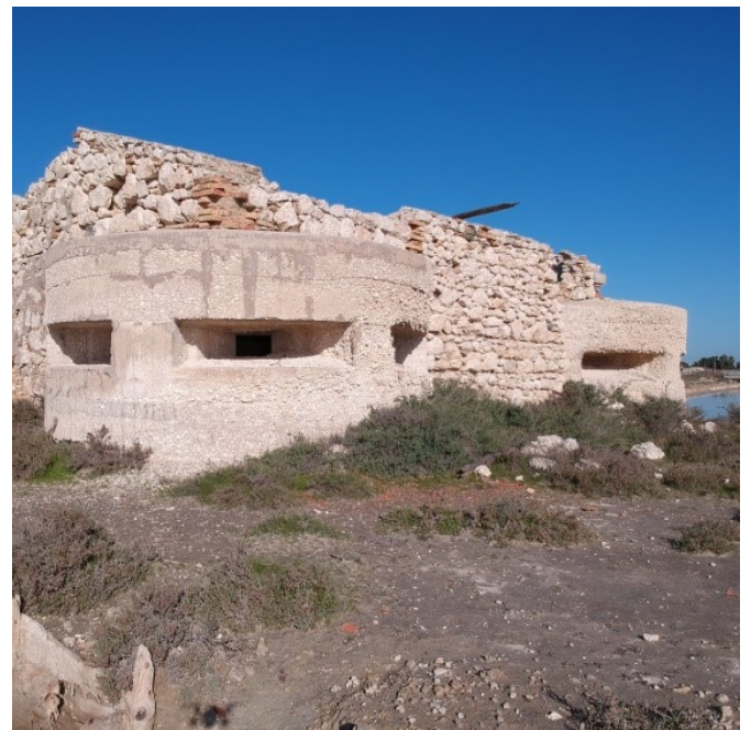
Figure 8. Sector 1. Bunker 1c: two bunkers inserted in a vernacular building (photo by N. Paba).
