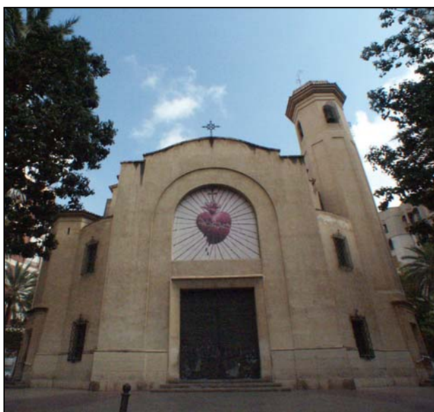
Figura 1. Fachada principal (Sur).
