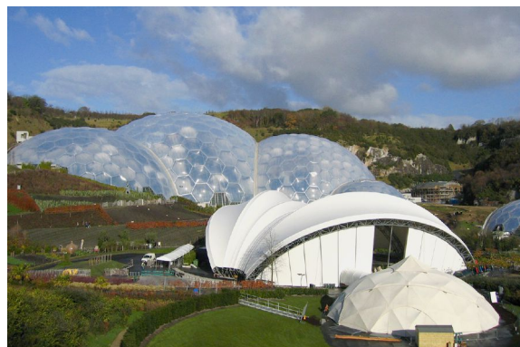
65. EDEN PROJECT ICE RINK STRUCTURE
