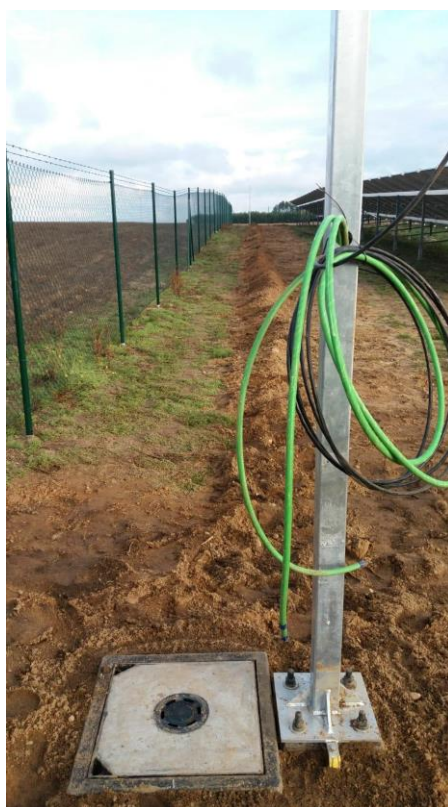
Image 62: Pole with cabling and a manhole after foundation works. [own photo]
