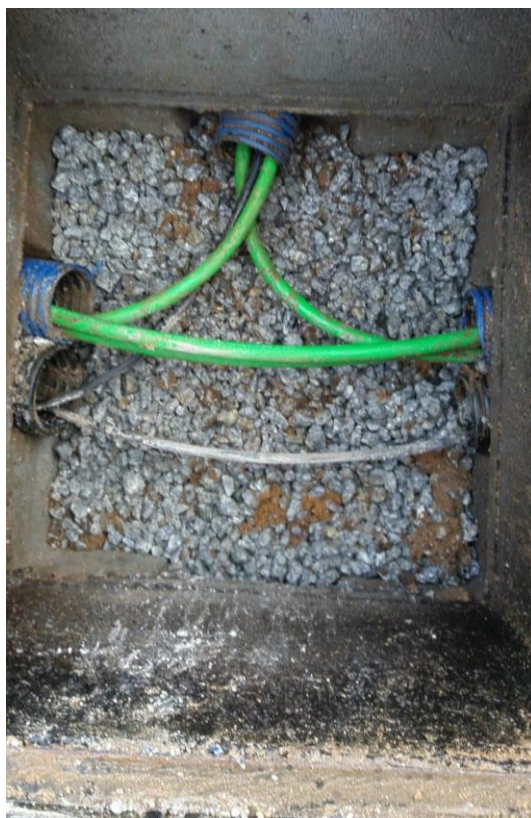
Image 61: CCTV foundation works. [own photo]
