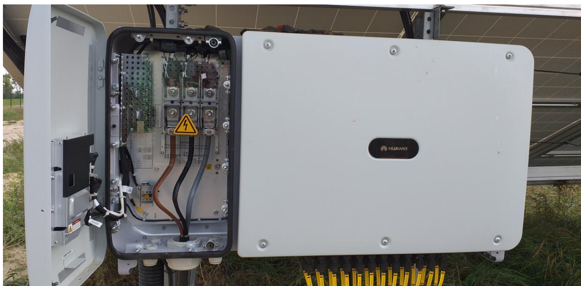
Image 29: Huawei Inverter for Lords project. In the left side, the 3-phase AC cable containing the monitoring signal. [own source]
