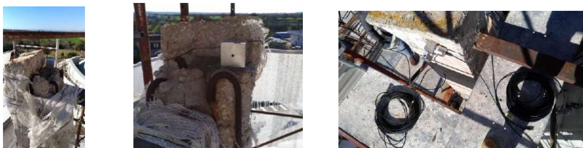
Figure 5. Details of the blocks placement and accelerometers connection
