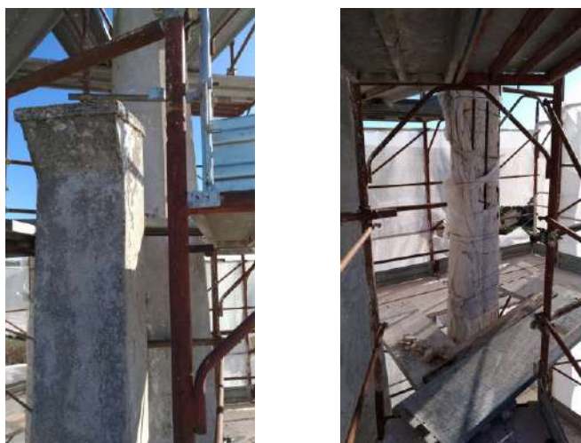
Figure 4. Details of coatings and scaffoldings before the retrofitting intervention.
