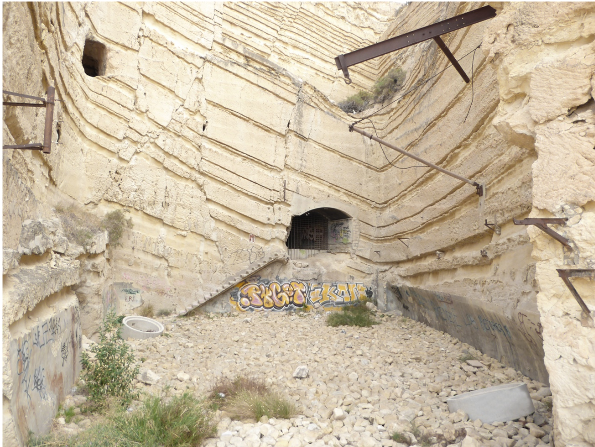
Figure 8. Image of the southern entrance to the complex, which was used as access to make the measurements taken from the stop of the TRAM de la Sangueta. It is trellised and in a deteriorated state such as the rest of the accesses (own source).
