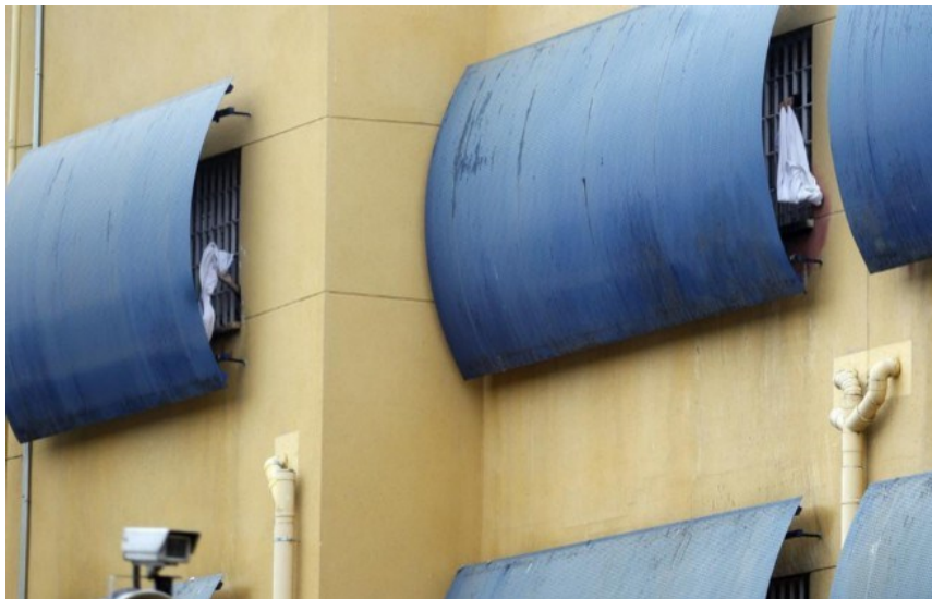
Figure 2. Blanket disposition on Aluche CIE façade. Madrid, 2010. Source: Arainfo.
