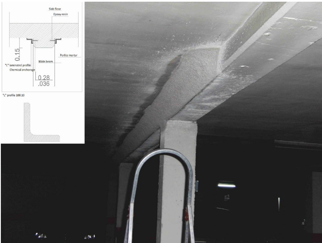
Figure 10. Detail of the steel angle reinforcements between the semi resistant joists and main beams.
