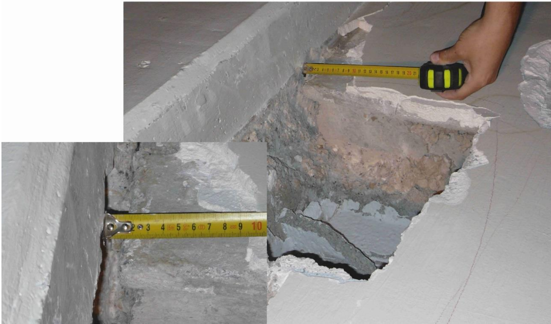
Figure 6. Inspection opening on the first-floor concrete slab (code CF-3 in Figure 1). A detachment of 1.3 cm between the semi resistant joist and the main beam was registered.
