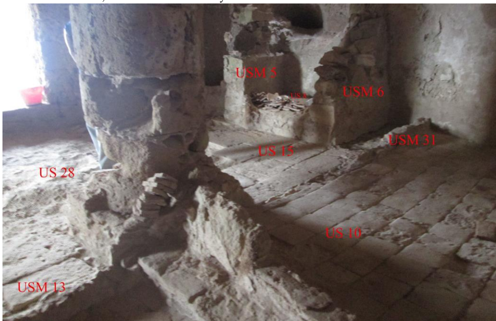
Fig. 11 – Capo Malfatano tower, USM and US into the round room (Maily Serra, 2014).
