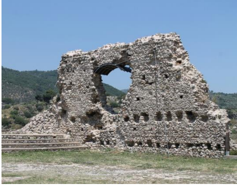
Fig. 9 Belcastro (CZ). The structure which supports the masonry above the heart-shaped gap.
