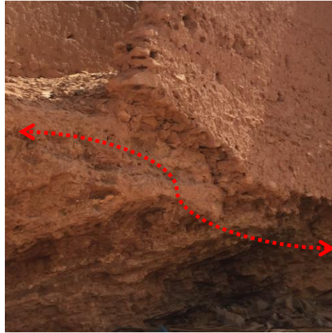
Fig. 13- Southwest wall stone constructive technique on the erected rock basement of Tala Aougrouit old fortress "El Guesba El Guedima" (Illili Mahrour, 2016)
