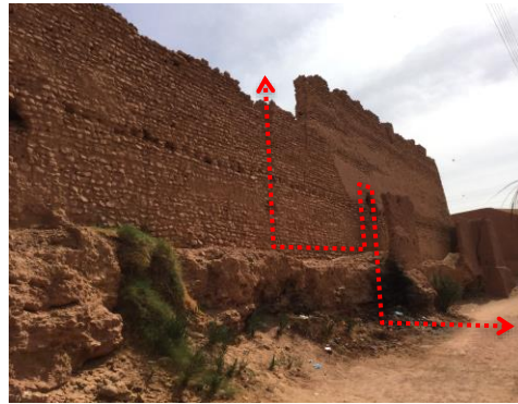
Fig. 8- Double walled west enclosure of Tala Aougrouit old fortress “El Guesba El Guedima” (Illili Mahrour, 2016)
