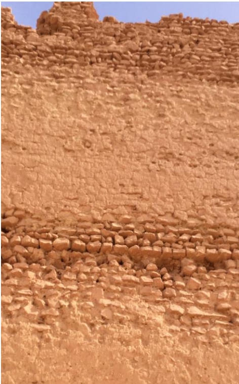
Fig. 12 - The wall regular stone layers of the western enclosure of Tala Aougrouit old fortress "El Guesba El Guedima" (Illili Mahrour, 2016)
