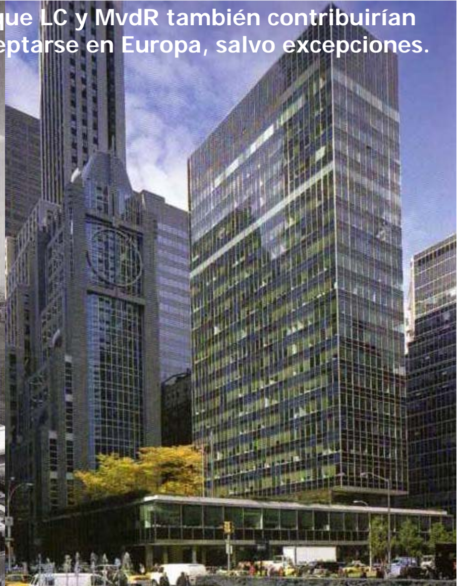
1950-52, Lever House , Nueva York, S.O.M. (Skidmore, Owings & Merrill)
