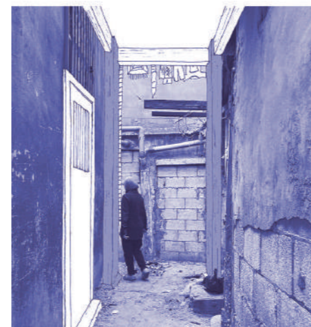
Fig. 7 - Minimal intervention through architecture.
