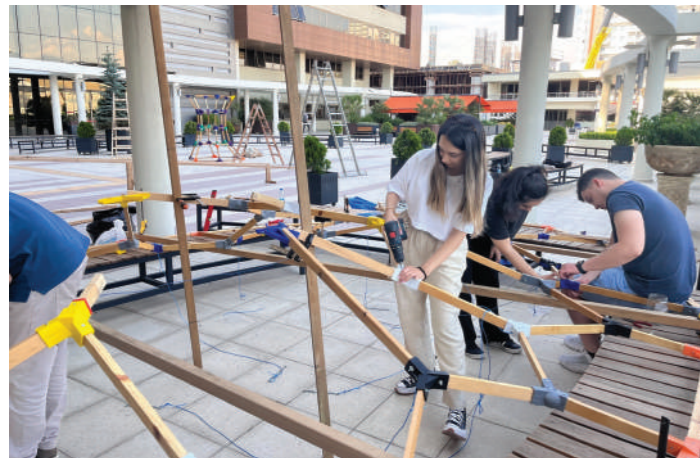
2. Assembly process of the canopy section.
