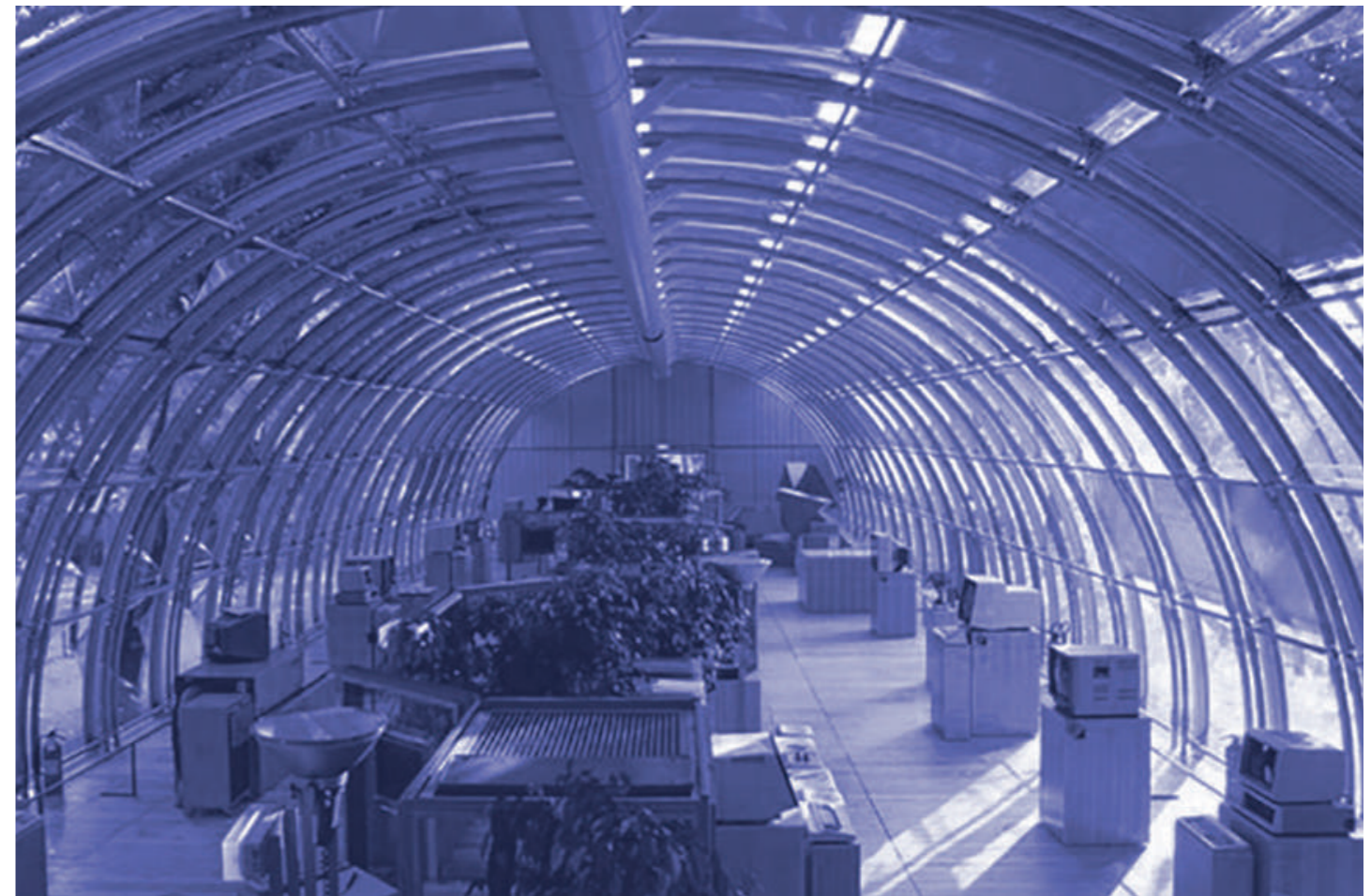
Fig. 1 - IBM Travelling Pavilion. Photo credit: Renzo Piano Building Workshop.
