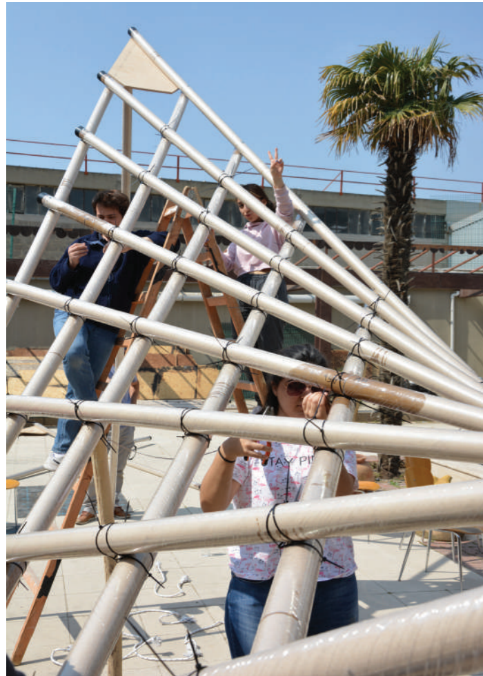
1. Assembly process of the structure.
