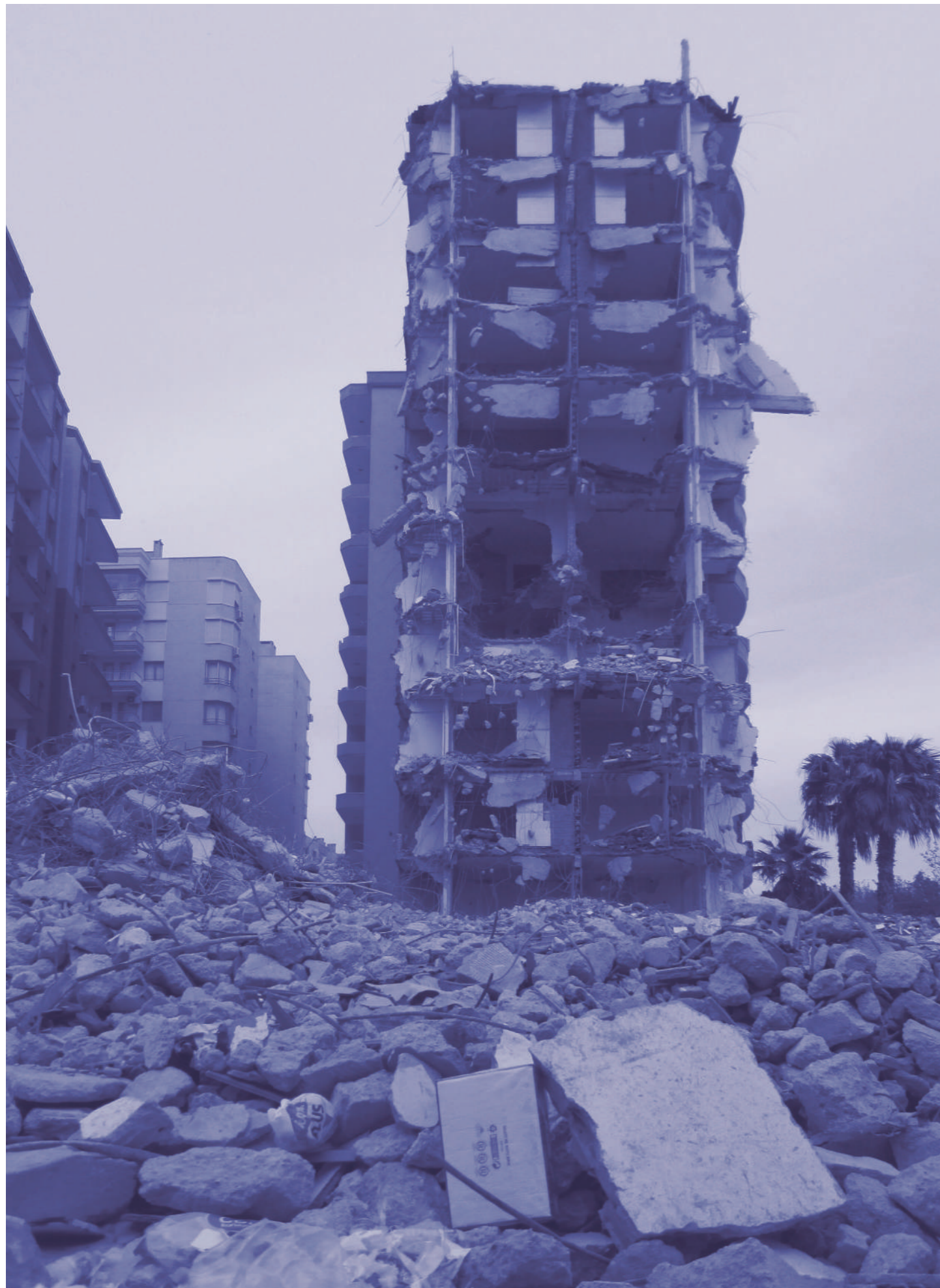
Demolition of buildings in Izmir..
