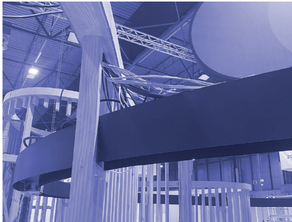
Fig. 9 - The black central ring as wiring distributor.
