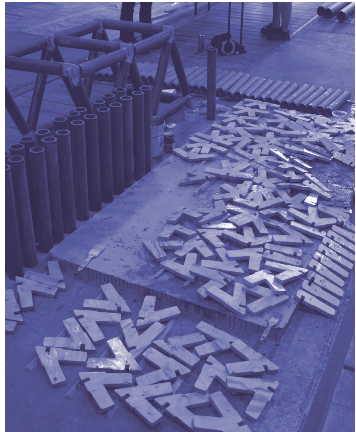
Components ready for assembly.
