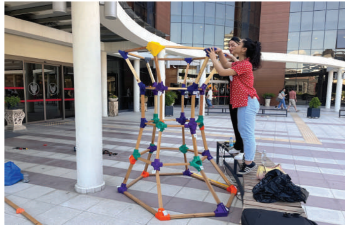
1. Assembly process of the column section.
