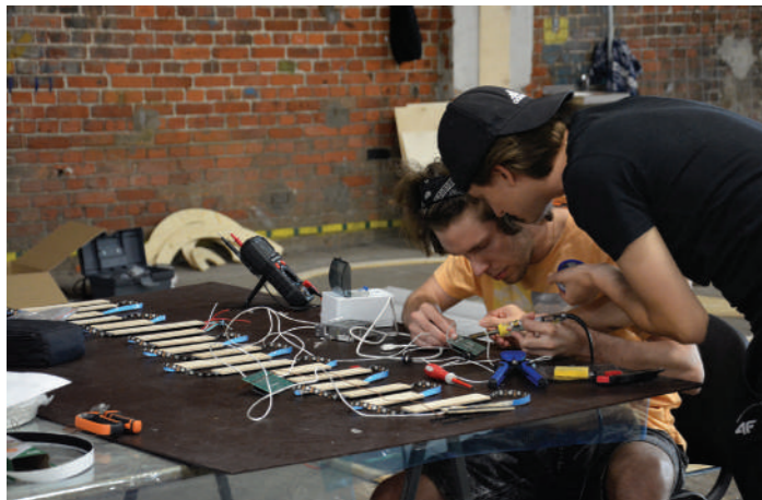
2. Electronic installation of the Reception Desk.
