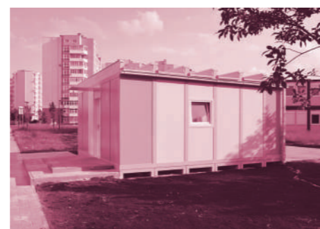
Styrofoam Housing System next to the relief container.
