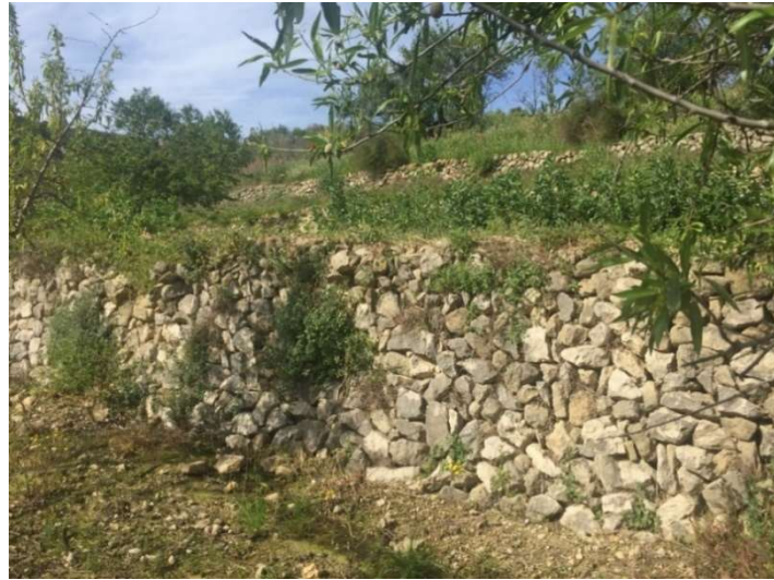
Figure 7. Slope terracing by dry stone walls for the almond trees cultivation.
