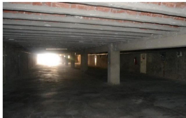
Figure 3. General view of building's basement.
