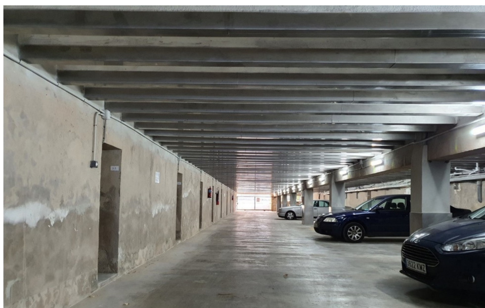
Figure 21. Final view of the finished repair work.
