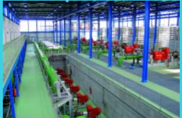
Fig. 11. Filtrated water pumping.
