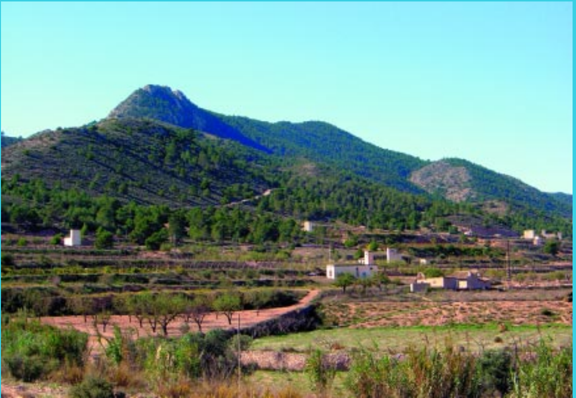
Fig. 23. Panoramic view of Barranco del Tolomó. Each of the towers corresponds to the location of the former electrical transformers and, thus, to the location of one or more pumping installations.
