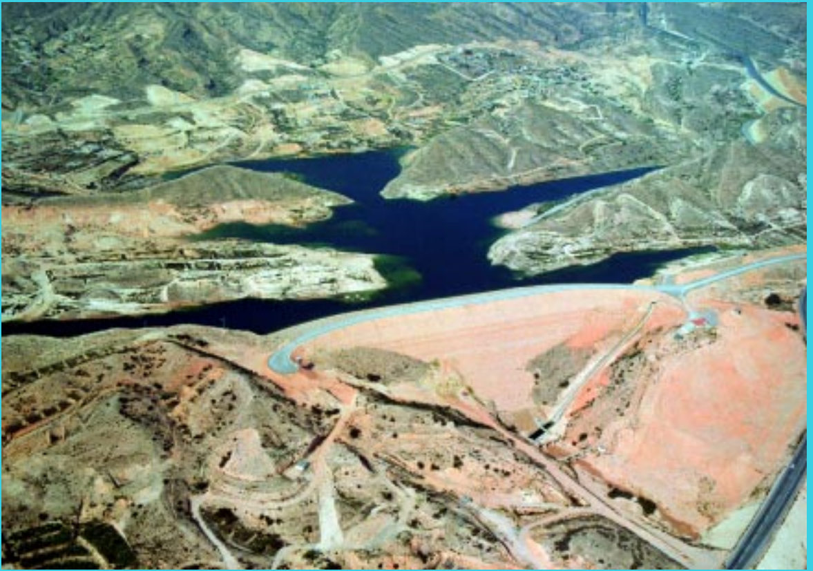
Fig. 15. Panoramic view of the Crevillente Reservoir.
