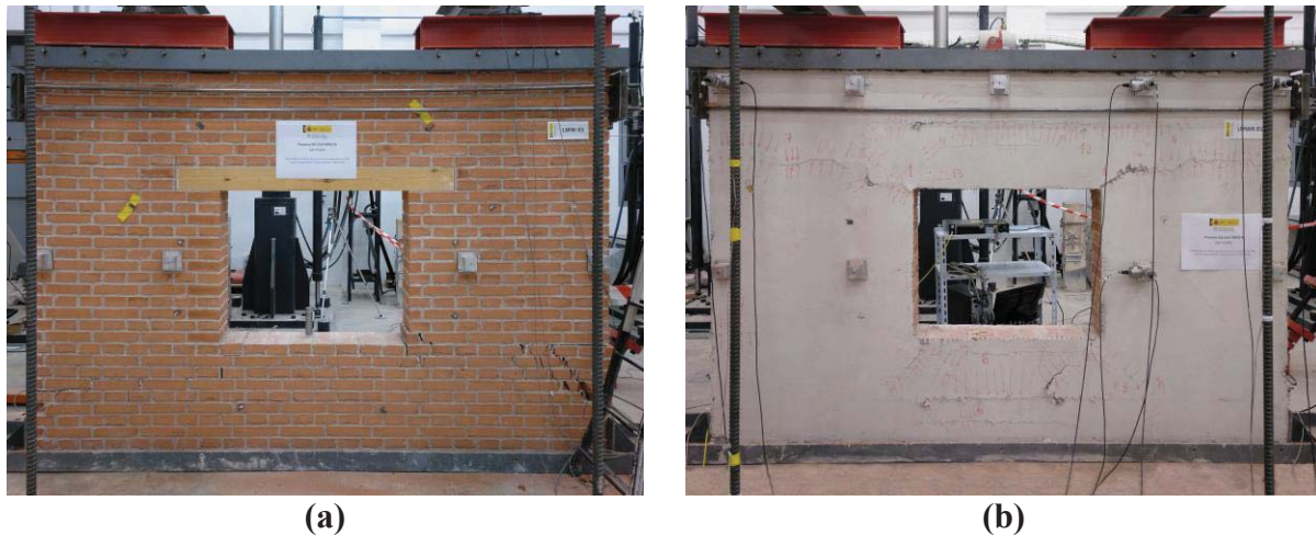
Figure 2: (a) Unreinforced and (b) reinforced masonry walls after damage.
