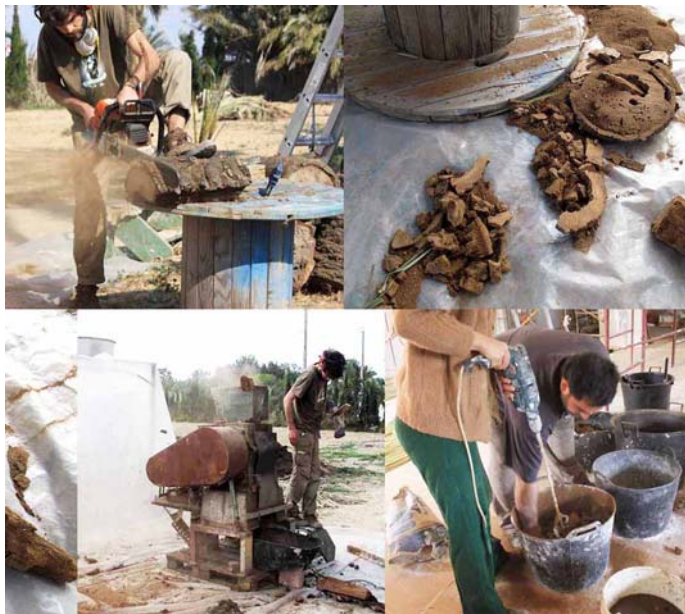
Figure 9. Roofing for Elche. External covering "Palmayola"
